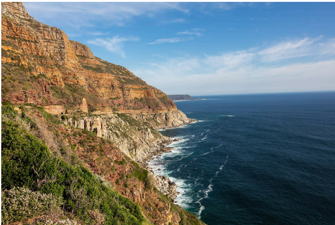
Chapman's Peak Drive – blasted into the cliff, a masterpiece of daring road building
